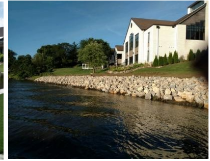
Shore Stabilization with Limestone Rip Rap wall
